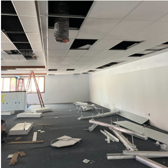
Removal of ceiling tiles and light fixtures
