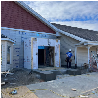
The new front entrance
