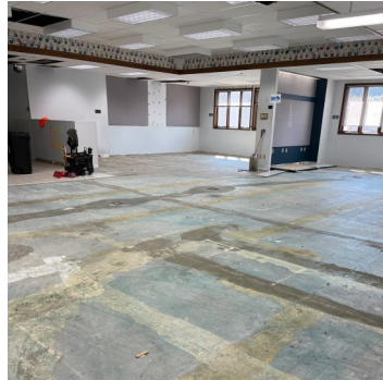
All flooring was replaced
