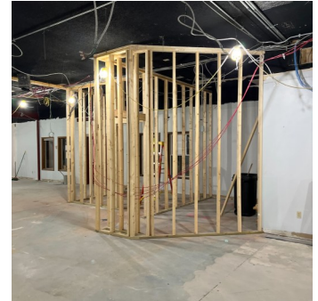
Construction of the 2 new private study rooms
